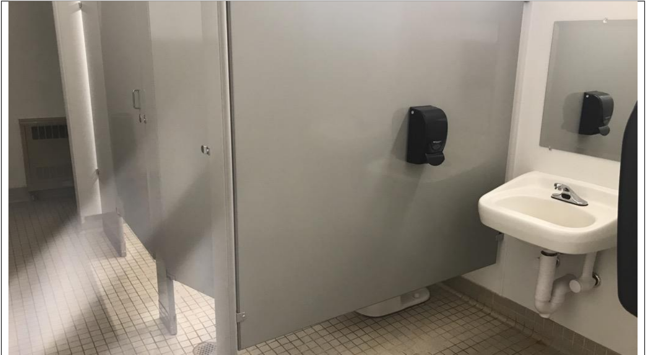
RESTROOMS HAVE BEEN REMODELED TO PROVIDE ADA STALL
