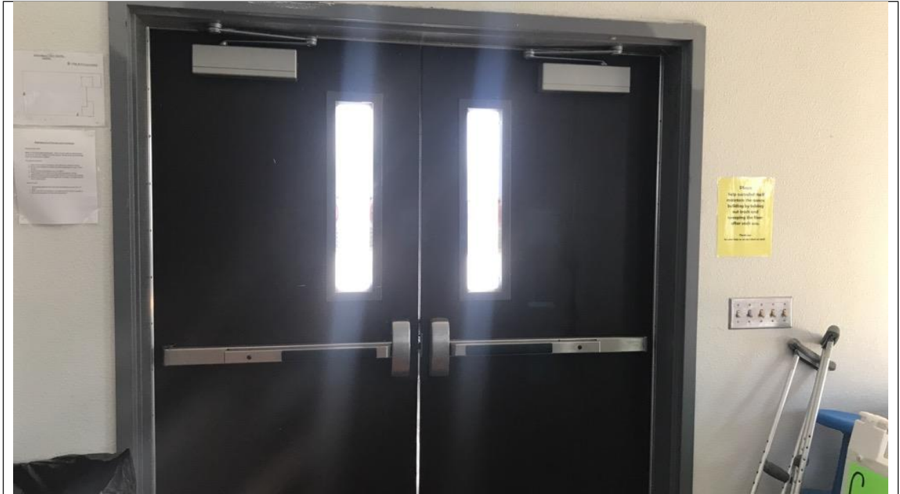
MAIN ENTRY / EXIT DOORS MEET ADA REQUIREMENTS
