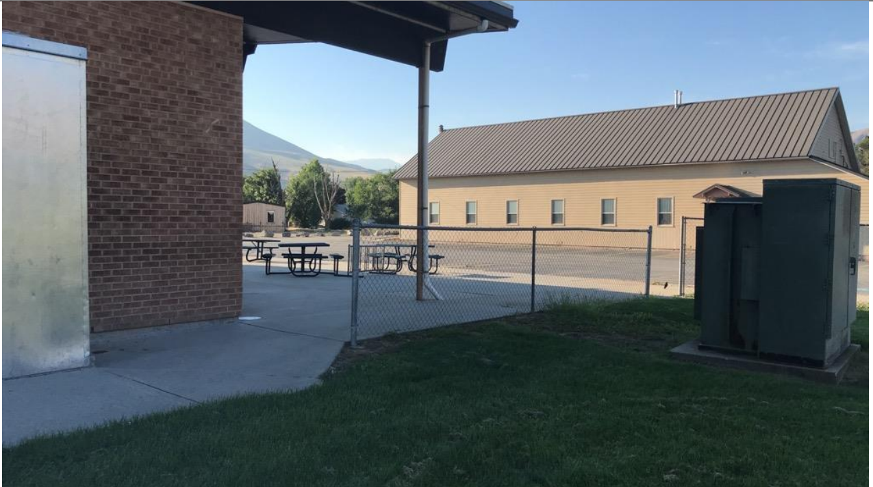
LOOKING SOUTH AT ANNEX AND EXTERIOR CAFETERIA AREA
