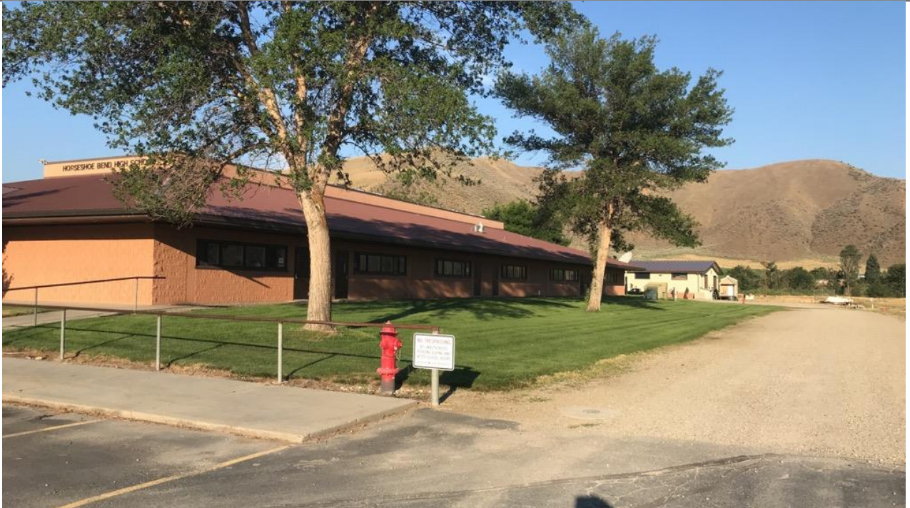
NORTHEAST CORNER / FIRE HYDRANT
