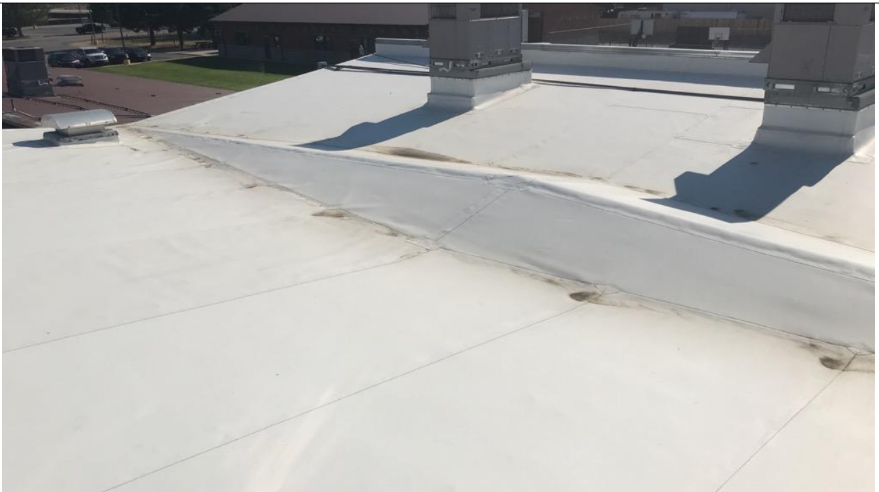
CRICKET AT LOW SLOPE ROOF TOWARD DRAIN TO LOWER METAL ROOF
