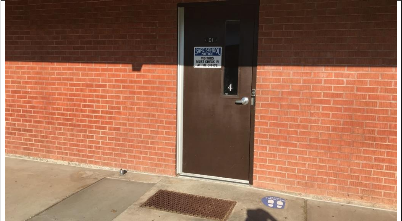
EXTERIOR DOORS WITH WALK OFF GRATES
