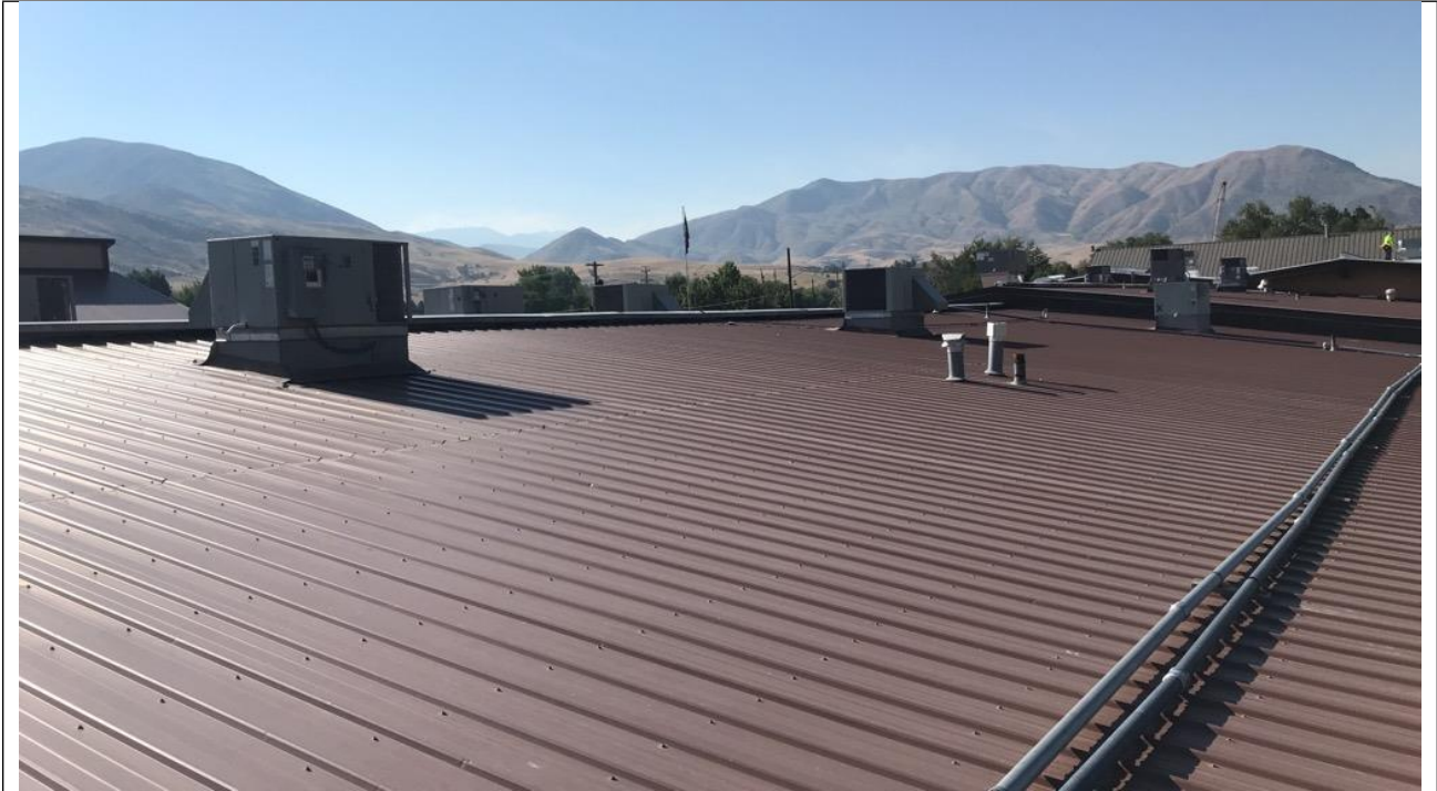
ELEMENTARY METAL ROOF AND HVAC UNITS
