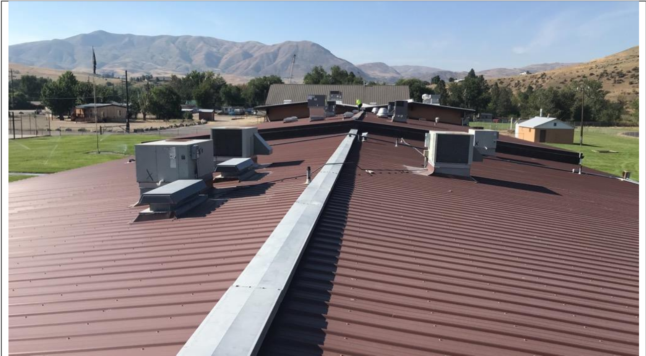
METAL ROOF / FAIR CONDITION
