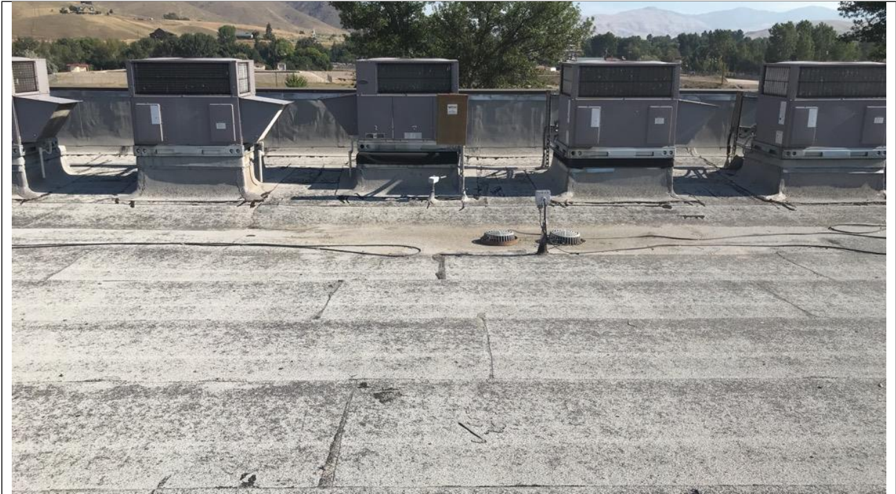
BUILT UP ROOFING SYSTEM AND ROOF TOP MOUNTED MECHANICAL UNITS
