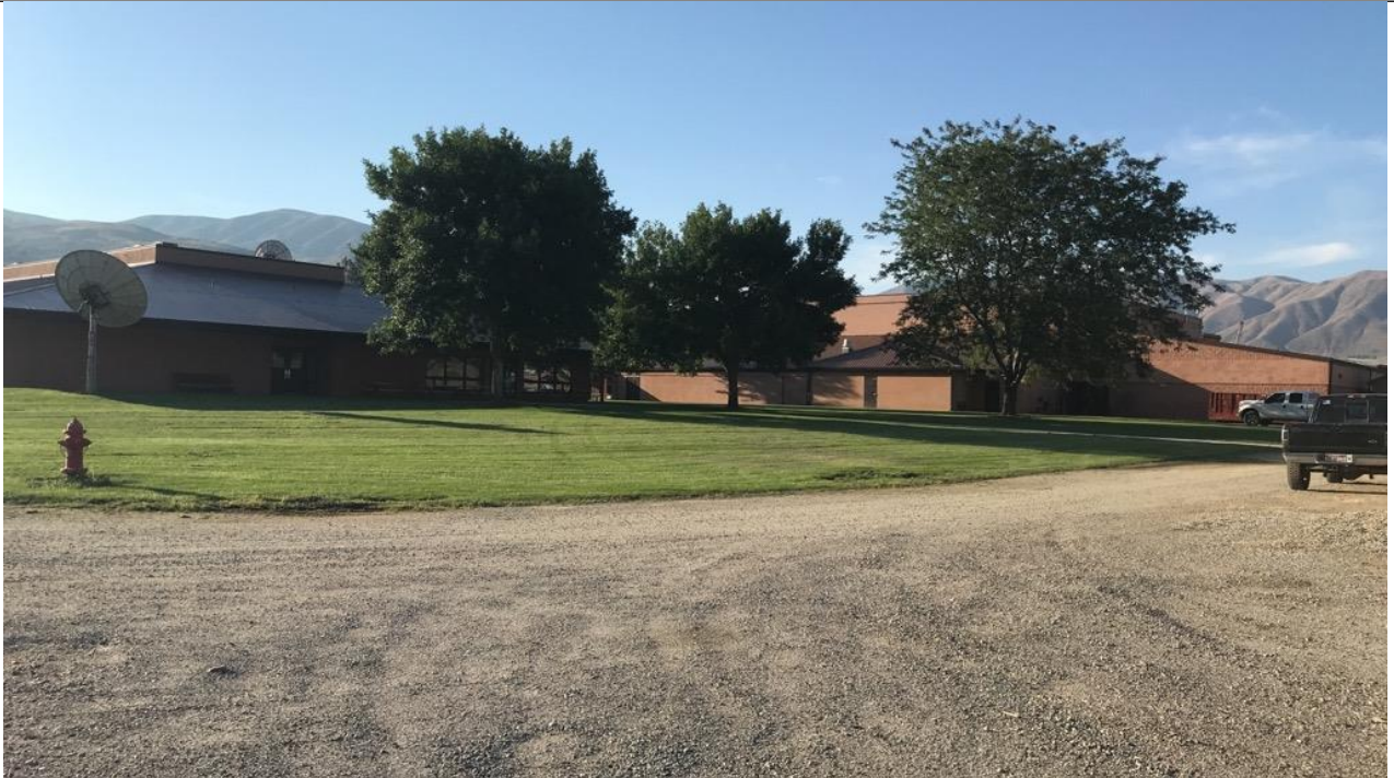
LOOKING EAST TOWARDS HIGH SCHOOL AND GYMNASIUM
