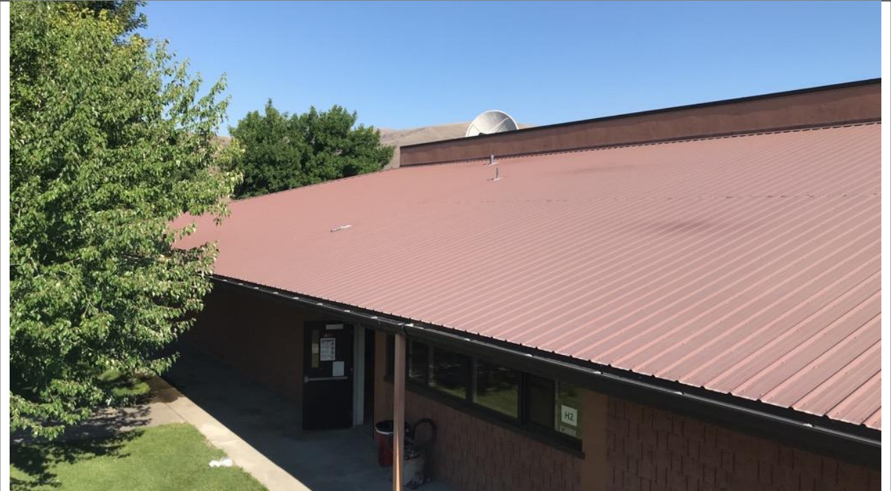
METAL ROOF AT ENTRY OVERHANG
