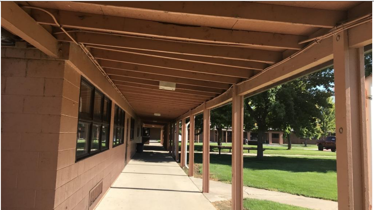
WALKWAY FROM ELEMENTARY TO GYM
