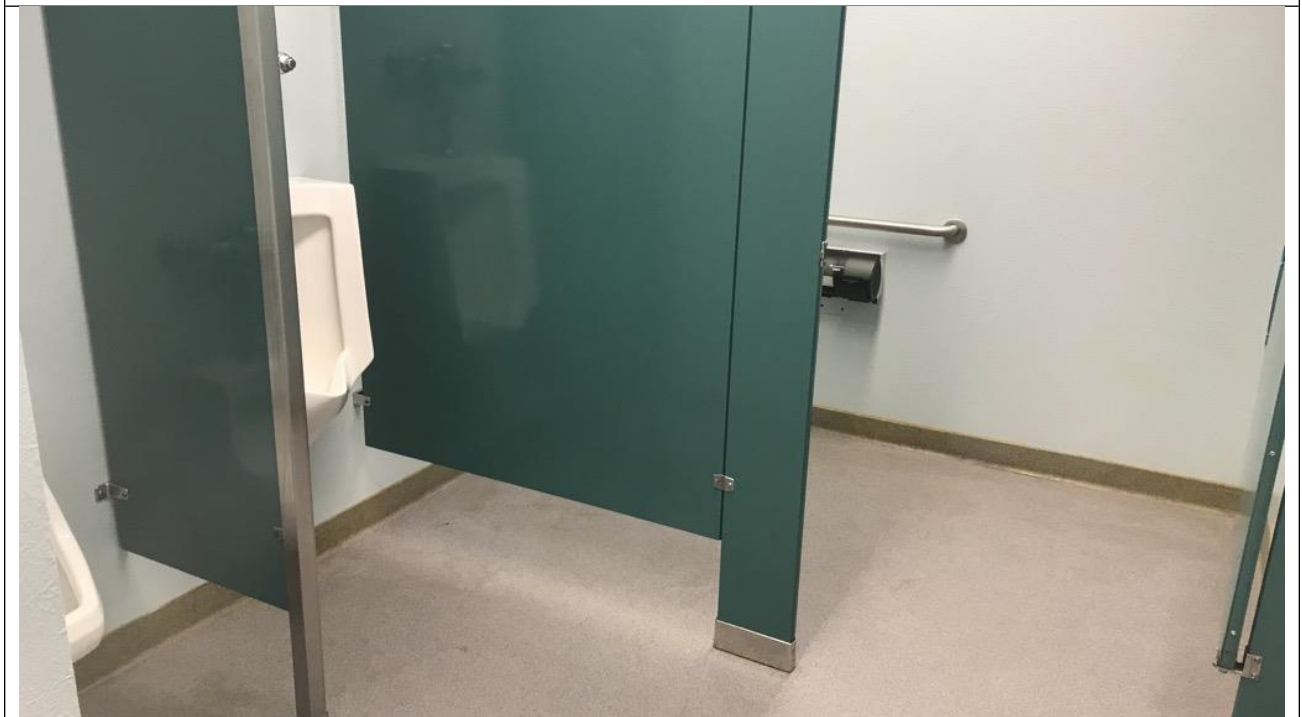
RESTROOMS / ADA COMPLIANT
