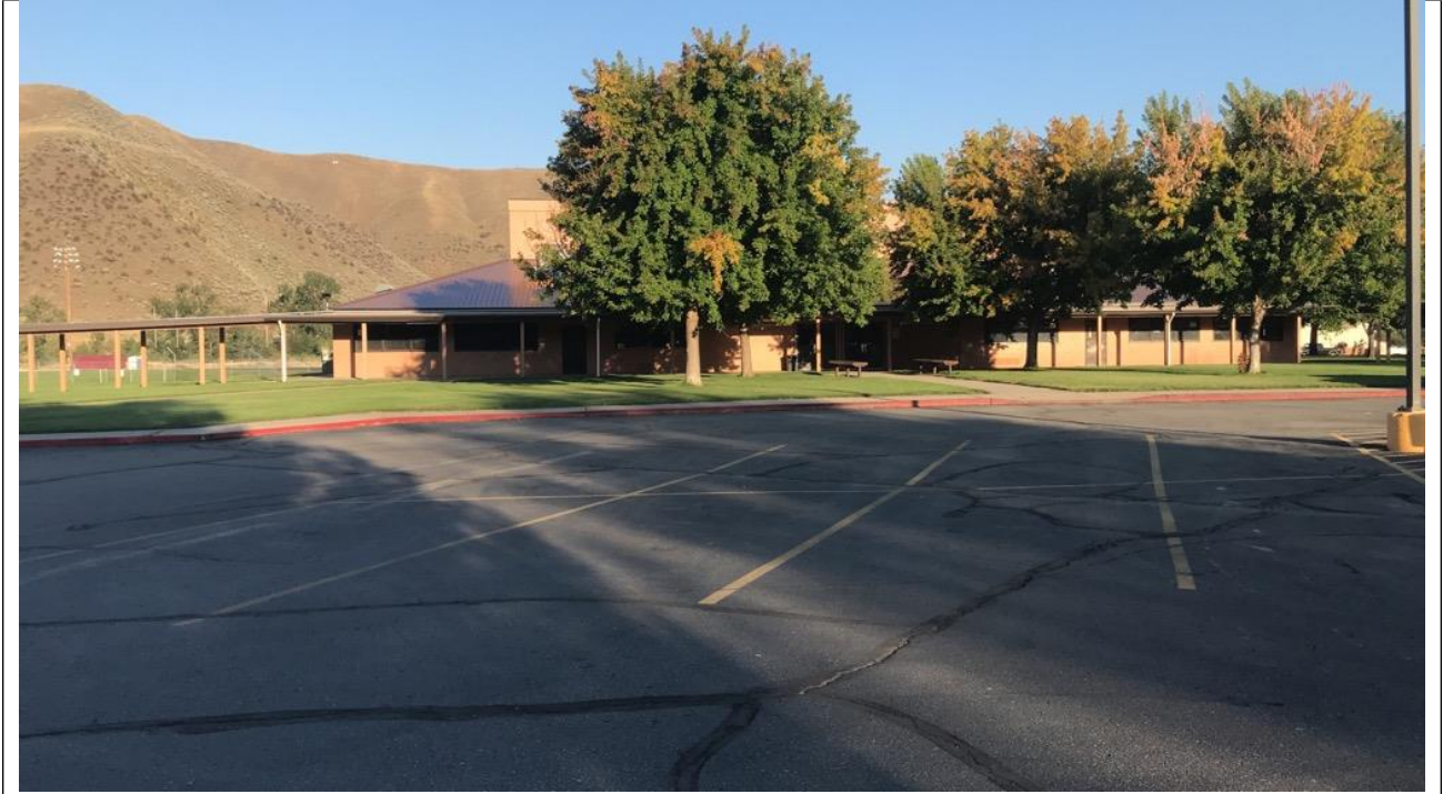
EAST FACING FRONT ENTRY
