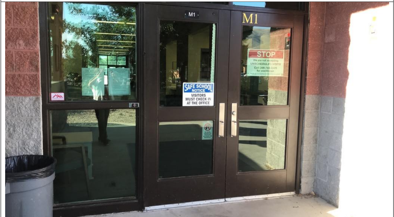
FRONT ENTRY DOORS
