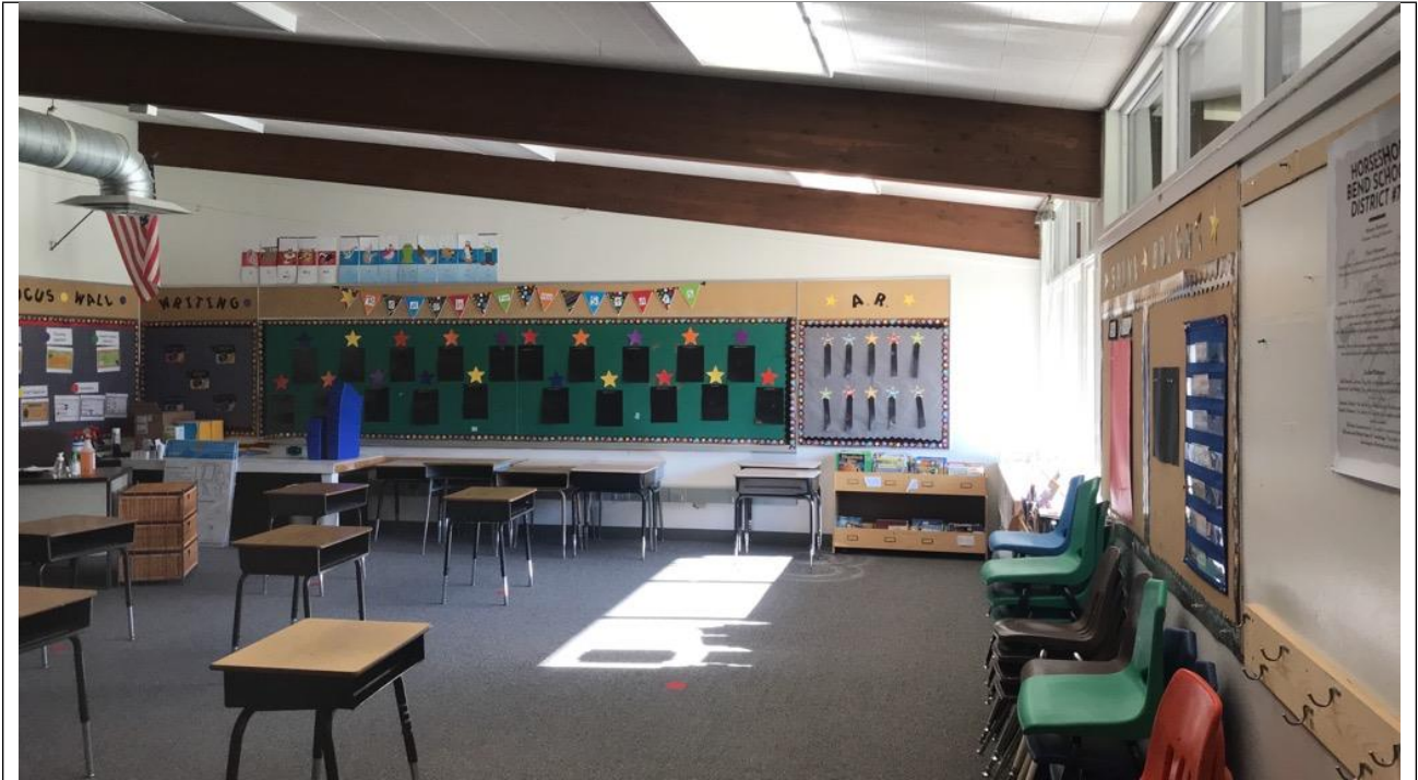
TYPICAL CLASSROOM – NO FIRE SPRINKLER SYSTEM
