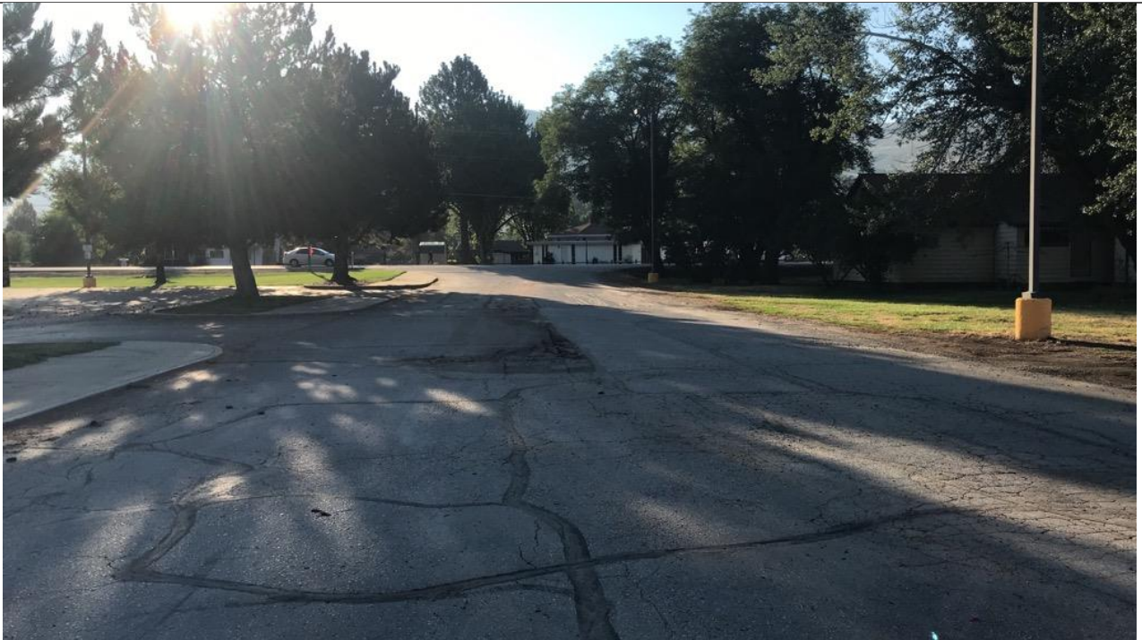
MAIN ACCESS DRIVEWAY LOOKING TOWARDS HIGHWAY 55
