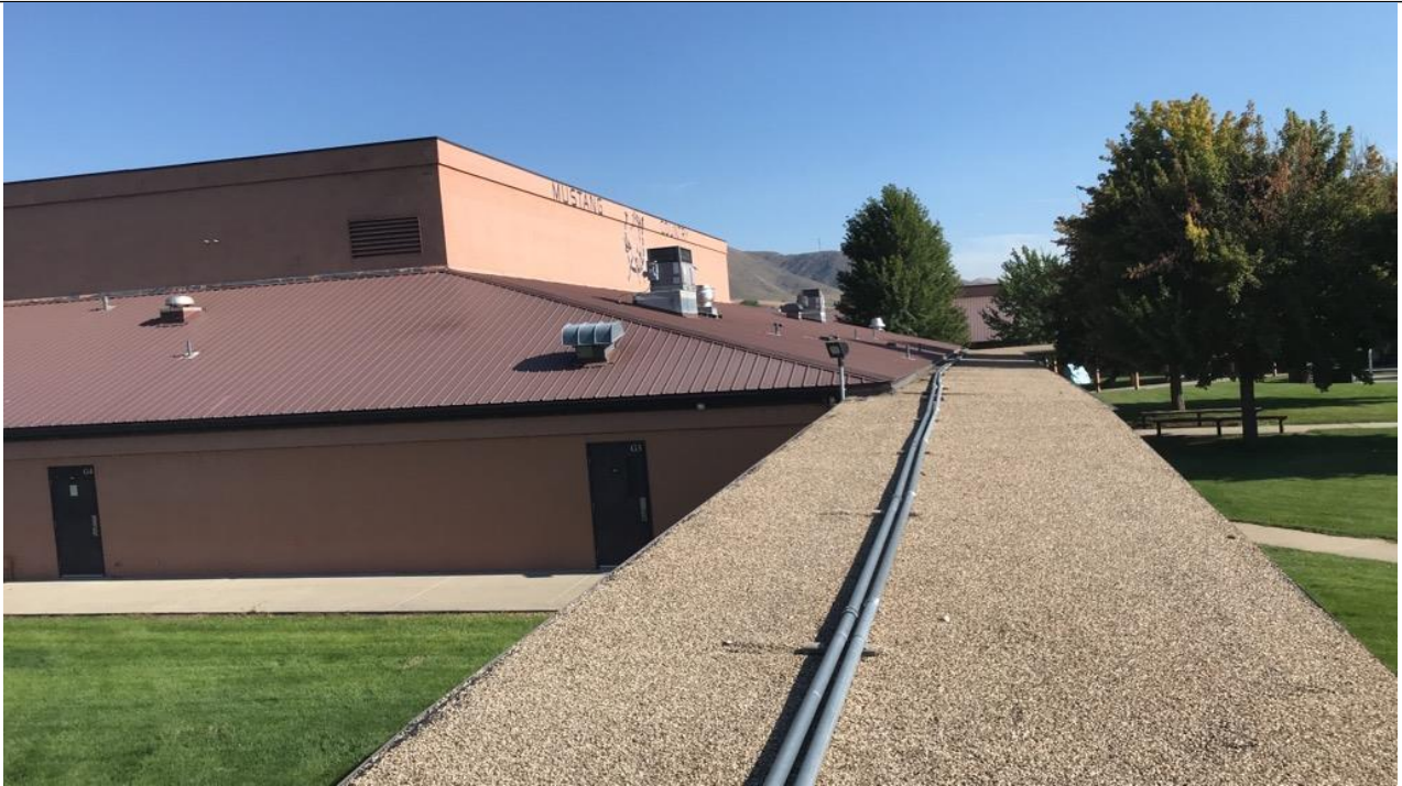
COVERED WALKWAY ROOF TOWARDS GYMNASIUM
