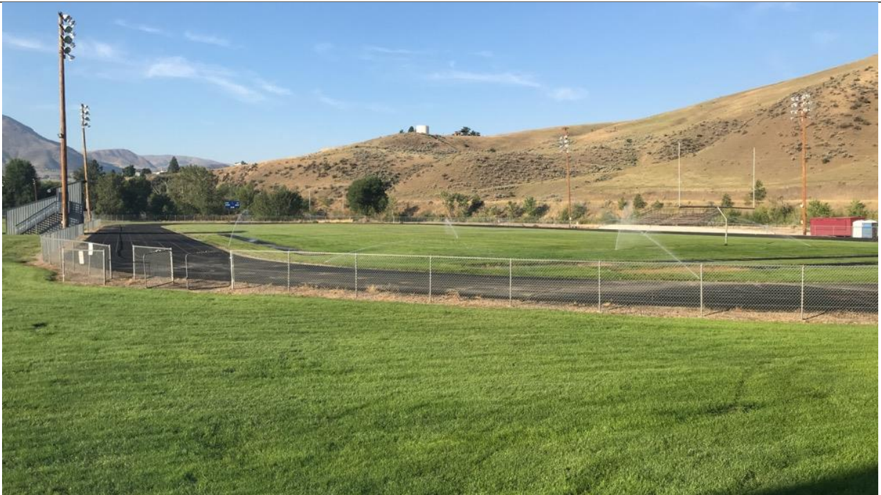
FOOTBALL FIELD AND TRACK. RUNNING TRACK IS IN POOR CONDITION
