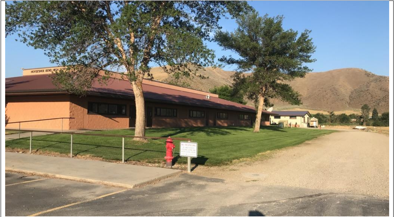
GRAVEL ACCESS DRIVE / HYDRANT AT THE NORTH OF HIGH SCHOOL
