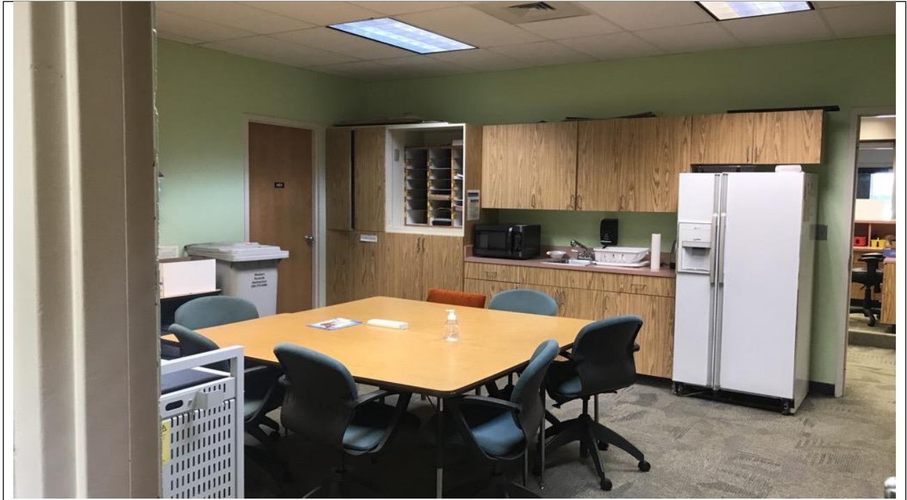
FACULTY ROOM / COUNTER HEIGHT DOES NOT MEET ADA REQUIREMENTS
