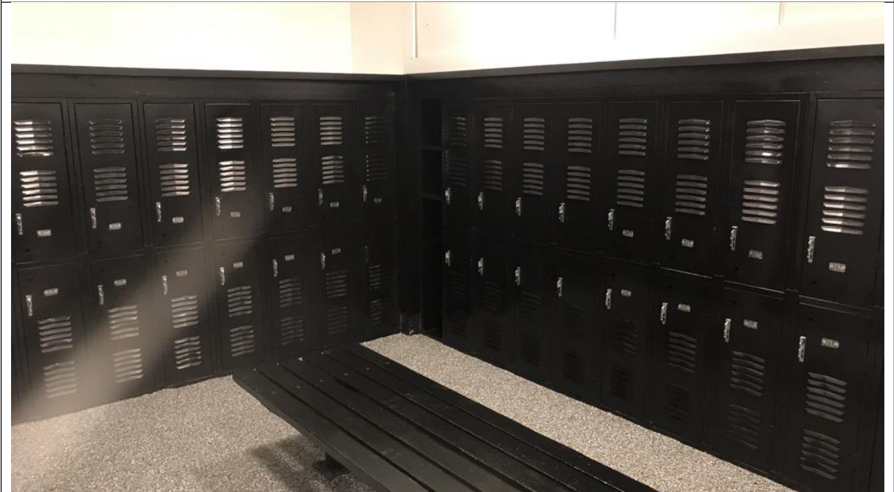
LOCKER ROOM / RECENTLY PAINTED
