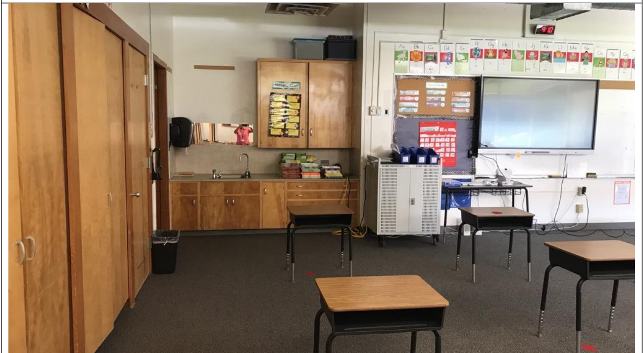
CABINETS ARE DATED. CLASSROOM TECHNOLOGY IS ALL SURFACED MOUNTED ELECTRICAL RACEWAYS
